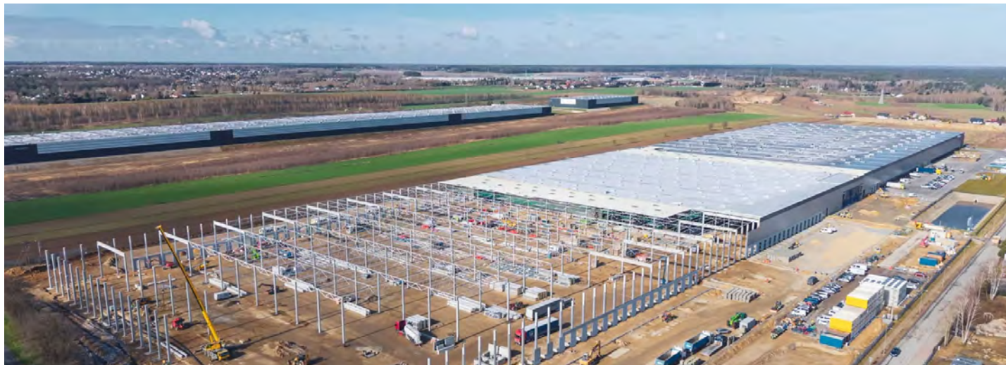
Bielenda's central warehouse (Łódź Voivodeship), source: Panattoni / press materials / panattonieurope.com
